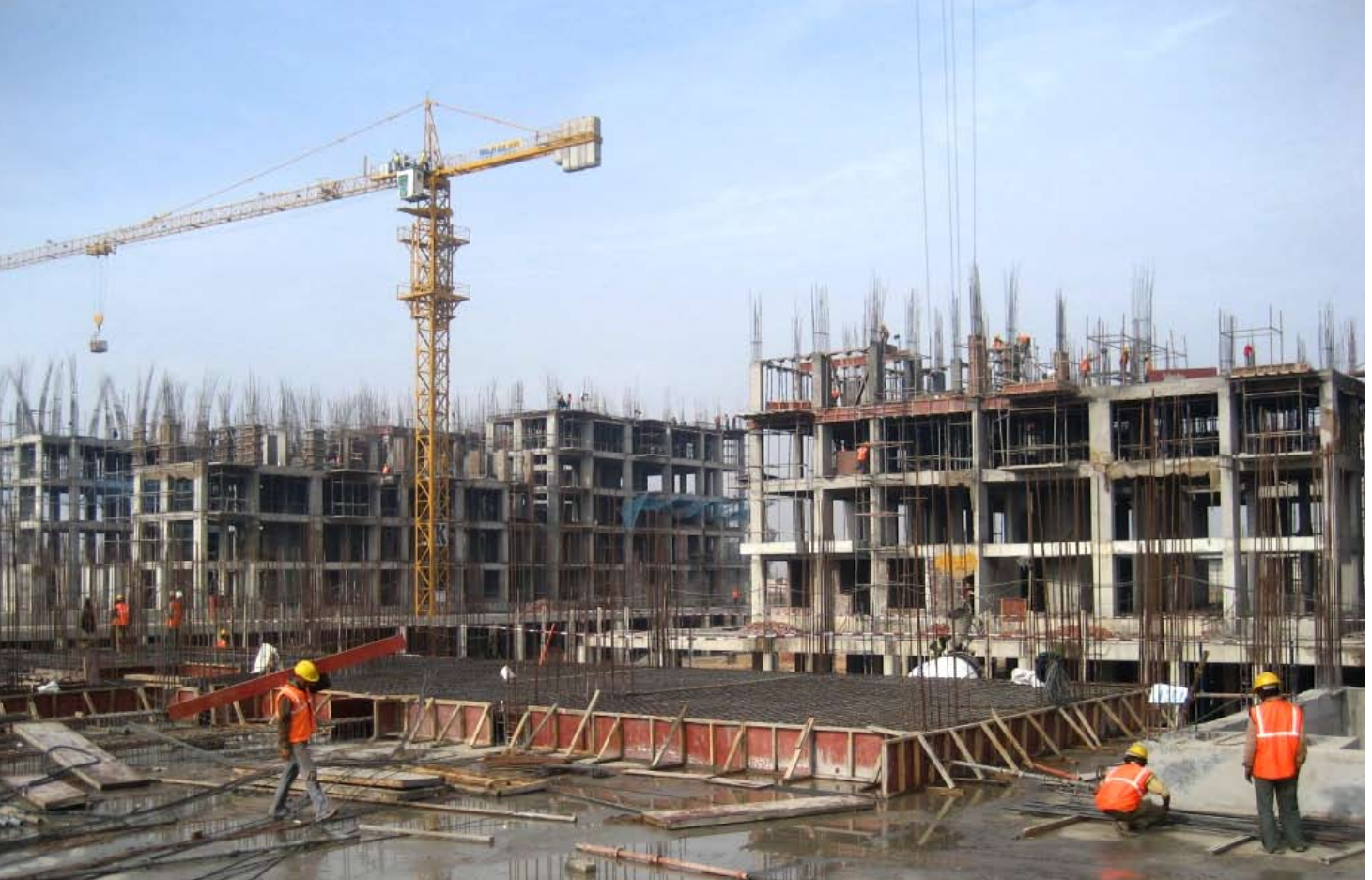
The Views construction in full swing
